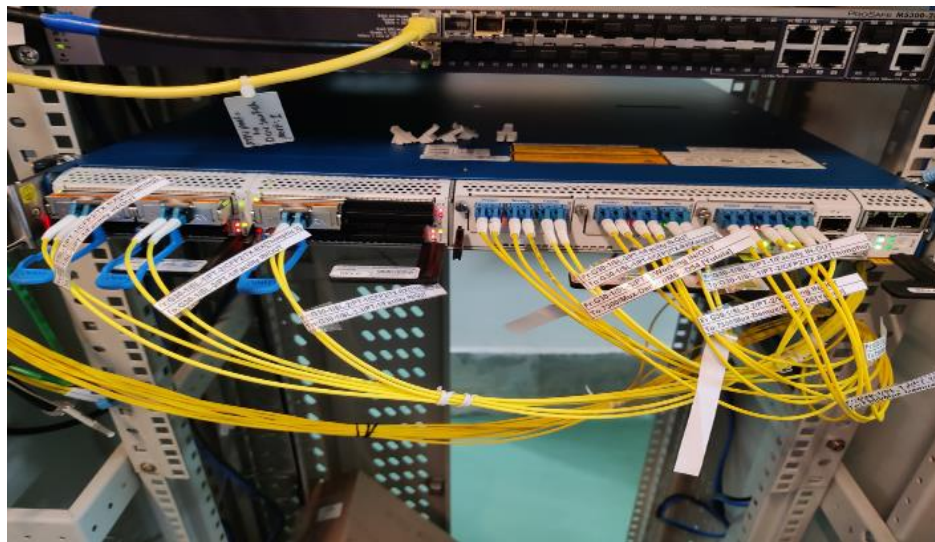
Figure 4: new IP DWDM installed at Jakar network center for IP DWDM connection to Thimphu and kanglung
